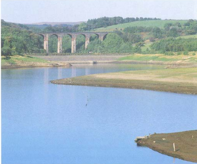
Wayott Reservoir in Lancashire. By controlling the frequency and degree of drawdown, viable wildlife habitats can be created.
